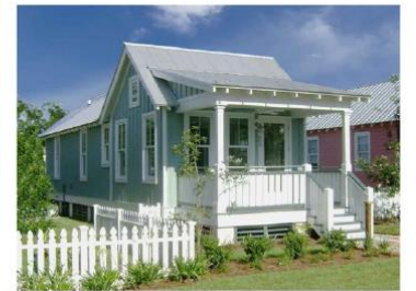
EXAMPLE OF MERIGOLD COTTAGE
