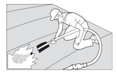
**Roof-top insulation:** Blowing fiberglass insulation through the roof top is effective at achieving good coverage and density on almost any metal roof. Use walk boards to avoid damaging the roof.
