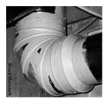
Sectioned elbows: Joints in sectioned elbows, known as gores, are usually leaky and require sealing with duct mastic.
