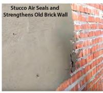
**Stucco over brick:** This retrofit serves two purposes: air sealing and structural reinforcement.
