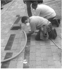
Blowing from the roof deck: Technicians remove a row of shingles, drill, and blow fiberglass into this vaulted roof cavity.
