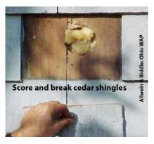
Score and break a shingle: If the shingles are flexible, you may be able to remove nails. However, usually you must score and break the shingle, and then later facenail it back in place.
