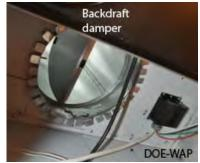
**Backdraft damper in the kitchen-fan housing:** Many kitchen fans have integral backdraft dampers.
