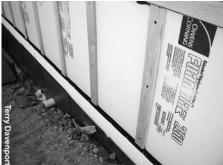
Foam sheathing with battens: Oneby-four battens are applied to 4 inches of foam board on the exterior to provide a fastening strip for siding and trim.
