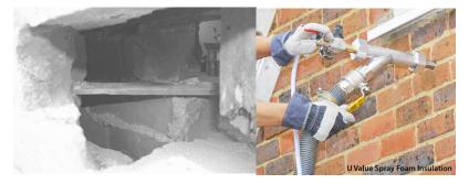
**Cavity brick wall:** Two separate single brick walls are held together by wood lath embedded in the mortar joint.
