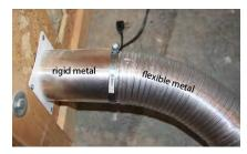
Vent and termination: Use rigid metal vent pipe if at all possible. Or use flexible metal vent and not foil vent when flexibility is required.
