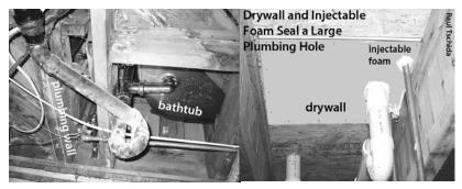
**Sealing large plumbing penetrations:** Bed drywall or wood sheathing in sealant and fasten with nails or screws. Fill gaps around the penetrations with one-part foam to complete this airtight seal.
