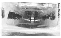
Lining a panned cavity: Foil-faced foam board, designed for lining cavities is sealed with duct mastic to provide an airtight return.
