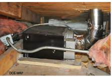
**Right-way fan orientation:** Air stream turns 90 degrees which is acceptable.
