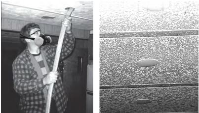
**Blowing through the ceiling:** The contractor pushes the fill-tube into the cavity and out near the edge of the roof. The holes are drilled in a straight line for appearance sake.
