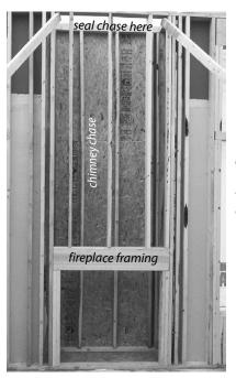
**Chimney chase:** Chimney chases can be multistory air-leak conduits if they're not sealed at floors and ceilings.
