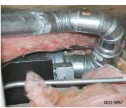
**Wrong-way fan orientation:** Turning the air stream 180 degrees substantially reduces airflow.
