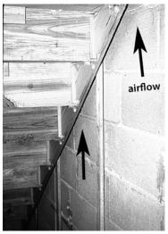
**Unfinished stairways:** Unfinished spaces underneath stairs create major air leakage pathways between floors and between the attic and crawl space or basement.
