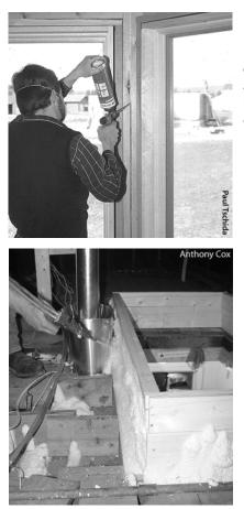
**One-part foam:** A contractor uses an applicator gun to seal spaces between framing members and around windows.
