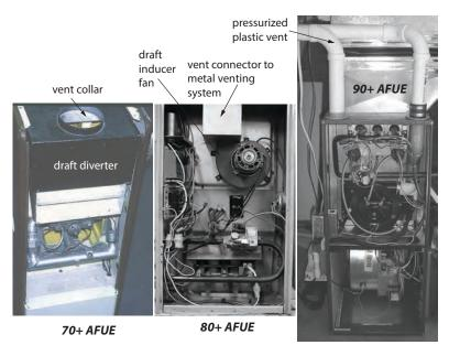
**Gas furnace evolution:** Energy auditors should be able to identify the 3 types of gas and propane furnaces. Only the 90+ AFUE furnace has a pressurized vent. The two earlier models vent into traditional natural-draft chimneys.
