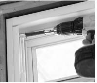
Block frame window installation: Block-frame windows don't have a fin. Installers use plates or screws to fasten the window to its opening.
