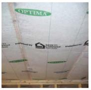
**Insulation restraint:** Workers patched access holes after they blew this floor through an air barrier.
