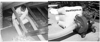
**Removing attic insulation:** Technicians vacuum and collect existing attic insulation for re-use or disposal because of moisture damage or to allow effective air sealing.
