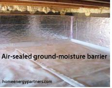
**Ground-moisture barrier:** An airtight ground-moisture barrier blocks water vapor and gases coming up from the ground.
