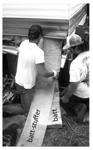
**Batt-stuffing walls:** Installers use a flexible plastic plank to stuff a fiberglass batt into an empty or partially filled wall cavity. Installers remove screws from the bottom of the siding. Joints between sheets usually remain locked together during batt-stuffing.
