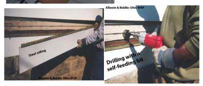
Remove the lower piece: Then drill holes for the insulation.
