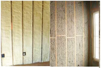
**Sprayed closed-cell foam:** Installers spray closed-cell foam short of filling the cavity or else they shave the excess off.
