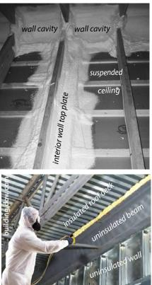
Sealing structural suspended ceilings: Two-part foam air seals and insulates an interior wall top plate and the wall cavity between the ceiling and roof deck.
