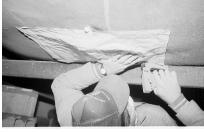
**Blowing a floor through the belly:** The contractor inserts a rigid fill tube through the belly to blow insulation into the floor cavity and underbelly.
