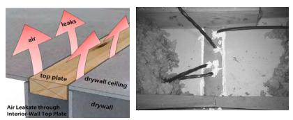
**Leaky top plates:** The cracks along top plates are from lumber shrinkage. They are small cracks but there are long lengths of them.
