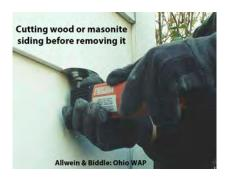
The last resort: When you can't find an easier way, cut horizontally the piece you want to remove. Re-install it after you insulate, and facenail it in place.
