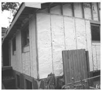
**Open-cell polyurethane foam:** The foam was sprayed into the cavities and the excess shaved off. New sheathing, house wrap, siding, and windows follow later.
