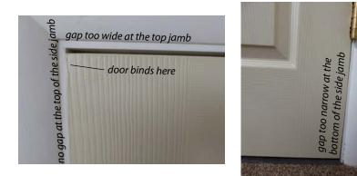
**Symptoms of a sagging door:** Gravity rotated this door to pinch the top jamb side corner and bottom hinge side corner of the door against the side jambs.
