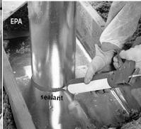
Sealing manufactured chimneys: When installing retrofit insulation in addition to air sealing, install a shield on top of the air seal that extends above the level of the new insulation.
