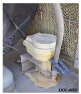
Float controls water supply: Make sure that the float shuts the water off completely when the reservoir is full.
