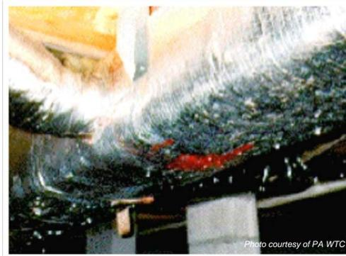
*Water droplets of condensation on AC ducts.*
